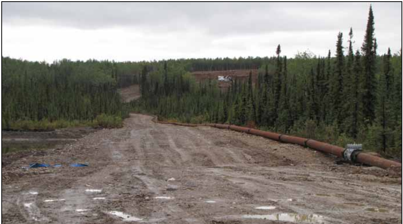
A view of the water line constructed from Clear Creek. The Big Alex bench and the wash plant is visible in the distance.
