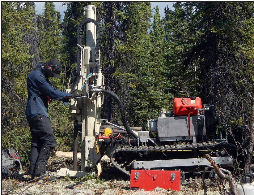
The rubber-track GTProbe vehicle operating in the field.
