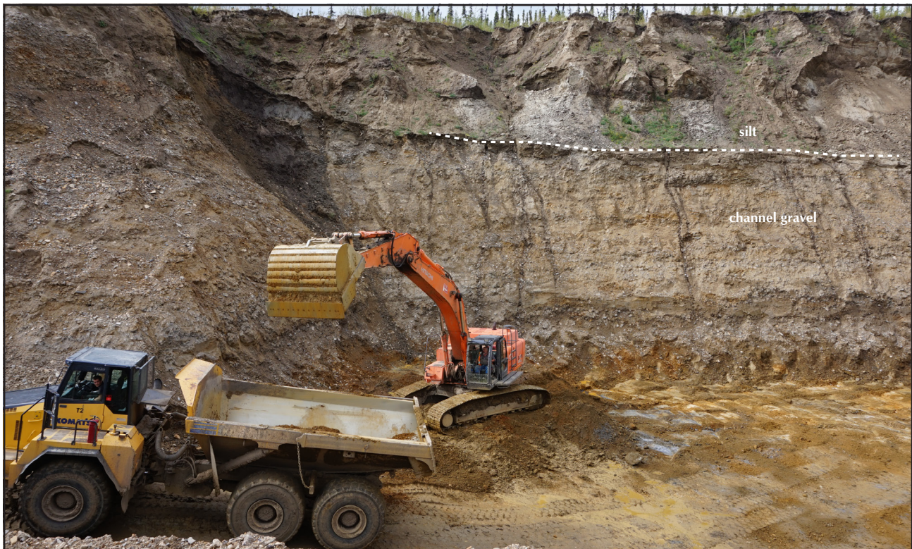
Figure 3. View of Fine Gold Resources 2015 pit on the left limit bench channel of Eureka Creek. The cut consists of 16.5 m (54 ft) of gravel overlain by 9 m (30 ft) of silt (loess). Both units are frozen. The bedrock surface continues to dip into the face and the full width of the channel has not been exposed.
