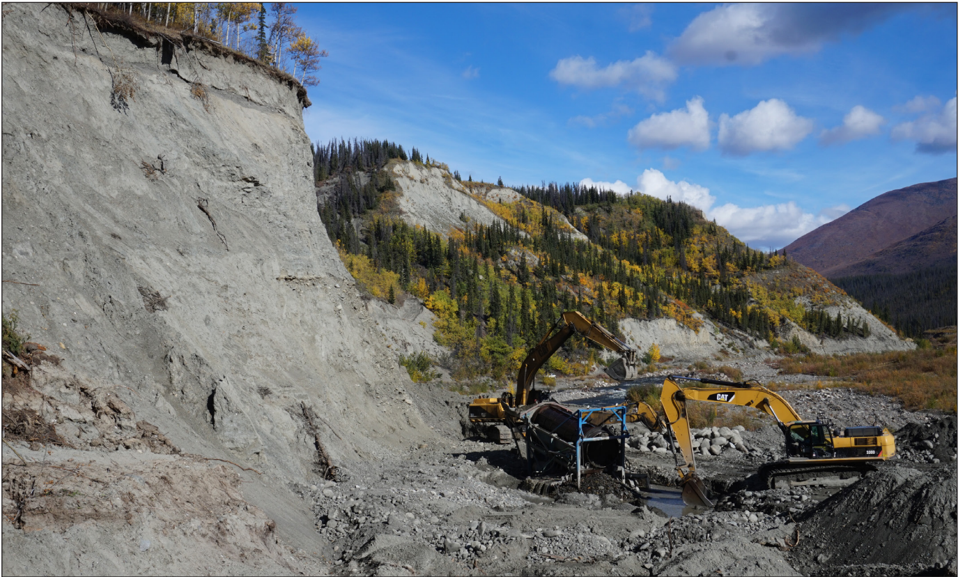
Figure 21. A view of the right limit excavation on Gladstone Creek. Mining efforts are focused in coarse gravel deposits overlying a compact till. Thick sequences of sediment are located above the excavation that contain past interglacial and glacial material.
