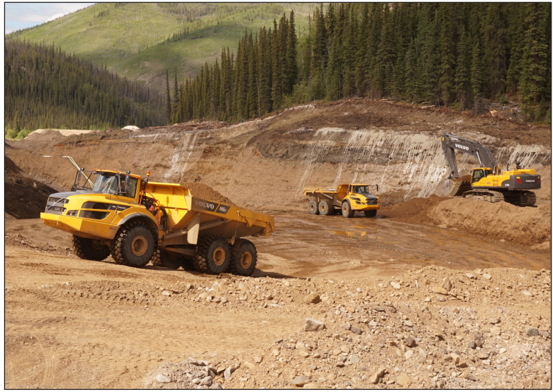
Figure 20. A view of the right limit deep channel pit on Seymour Creek in 2016.
