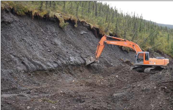
Figure 15. A view of the right limit bank on upper Glacier Creek. K-1 Mining is excavating the pay streak under colluviated weathered bedrock and muck.
