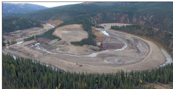
A view to the SE of Bear Roast Flat under active reclamation. The mine area at the left of the photograph has been contoured and top-coated, together with the drainage channel and settling pond
