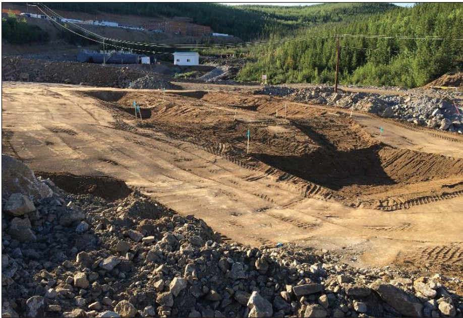
Demonstration scale CTWS foundation during construction.
