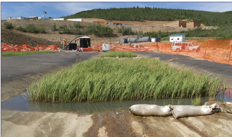
Plant establishment in the demonstration scale CTWS in July 2017.
