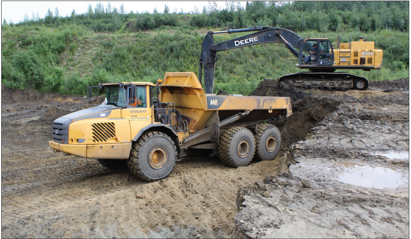
Figure 6. T.D. Oilfields reworking former dredged ground on lower Gold Run Creek. The seagull on the hood of the haul truck was a permanent partner at the mine this year, enjoying heated flooring and a free lunch.
