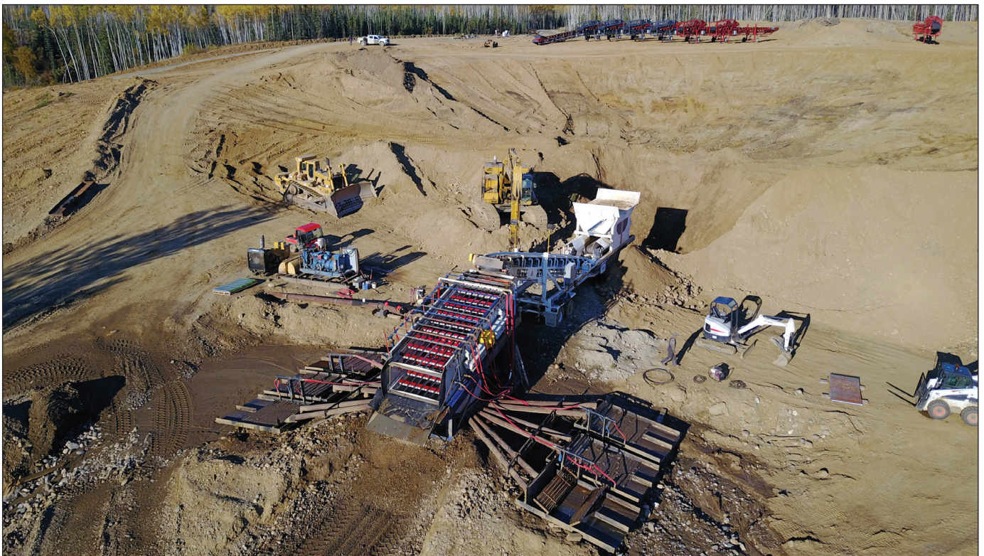
Figure 6. A view of the new wash plant and feeder being installed on Wolfhead Discovery and Mining's operation on lower Clear Creek.
