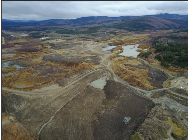
Figure 4. Aerial view of the mouth of Eureka Creek where Fine Gold Resources undertook a substantial reclamation project that involved surface grading and top-coating of legacy placer mine workings.
