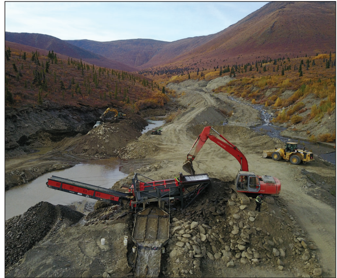
Figure 18. A view looking upstream on Fourth of July Creek of FTG Placers operation. Active excavation is visible on the left hand side of the valley bottom (right limit).
