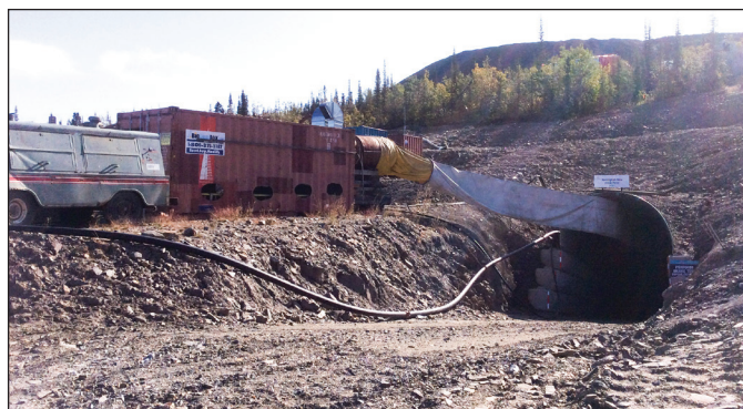
Figure 6. Bermingham mine portal.
