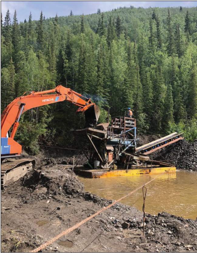
Figure 14. Fortymile Placers floating trommel plant on Marten Creek. One crew member operates a series of winches that swivel the plant and control the tailings stacker.
