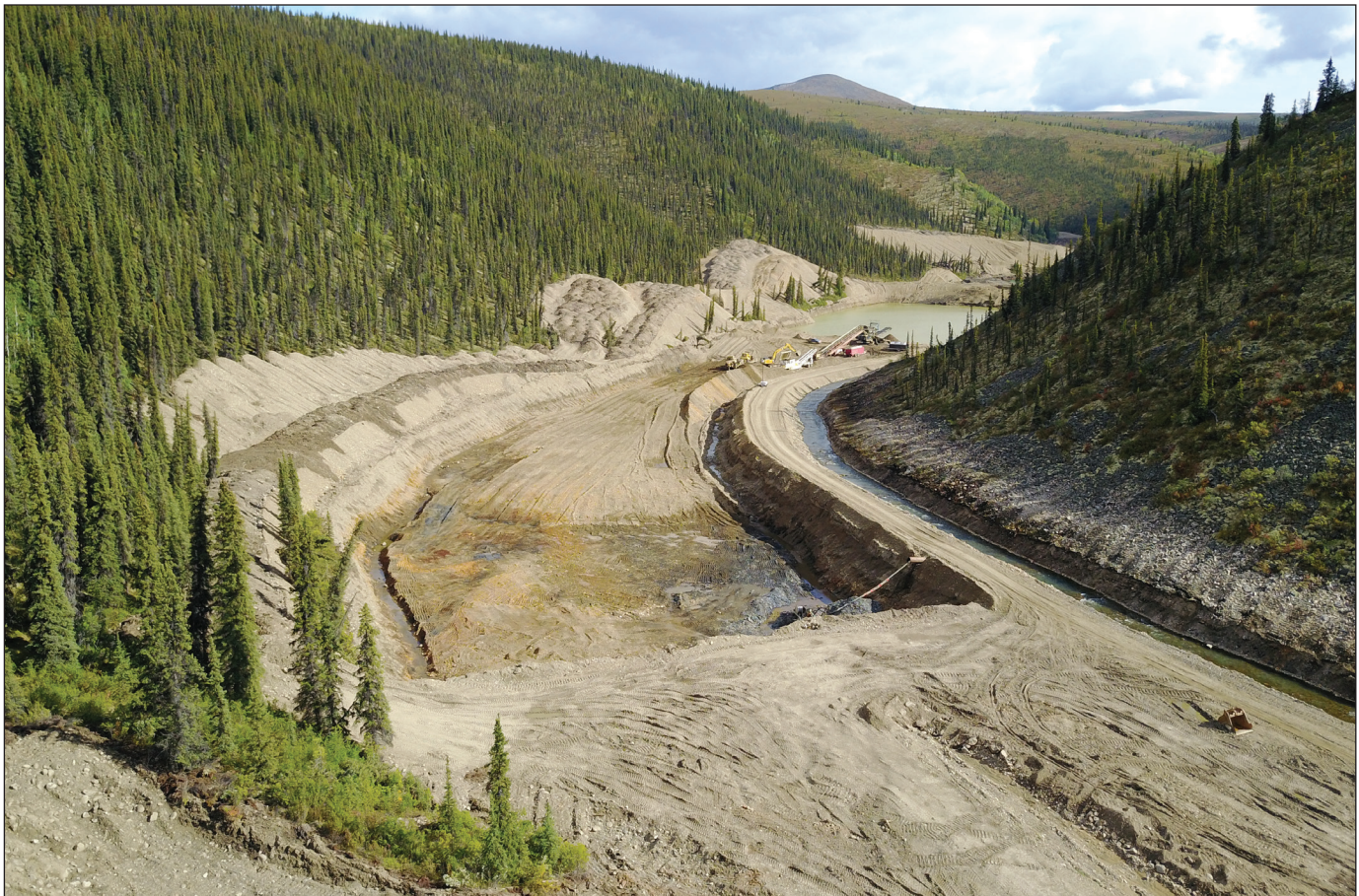
Figure 16. A view looking up Big Creek at Schmidt Mining Corporation's placer mine. In this section of the drainage the total gravel thickness is 5.2 m and a distinct high-energy, oxidized gravel measuring 2.8 m in thickness is present on bedrock and contains most of the placer gold.
