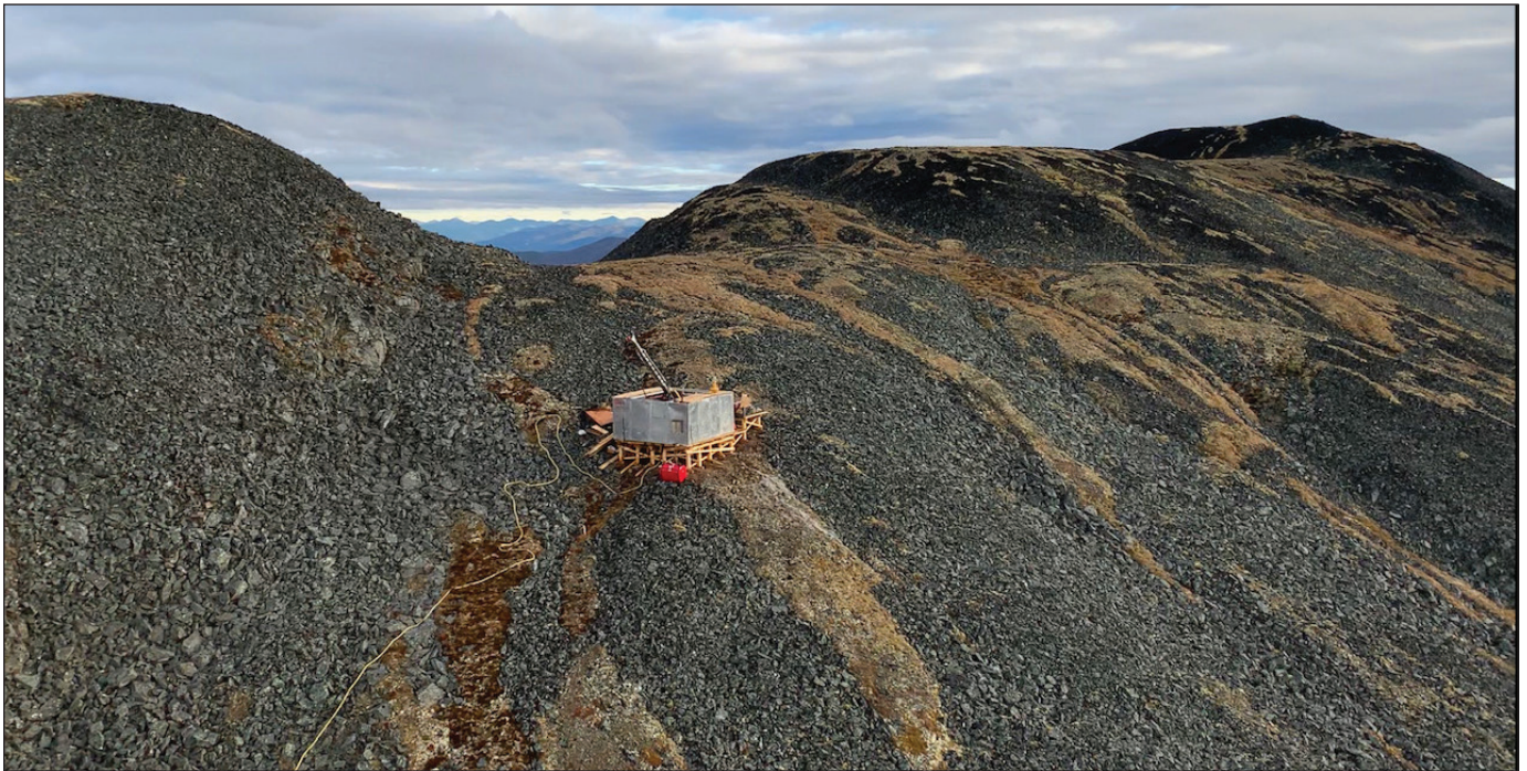
Figure 7. Drill rig at Sitka Gold Corp's RC property. Photo courtesy of Sitka Gold.
