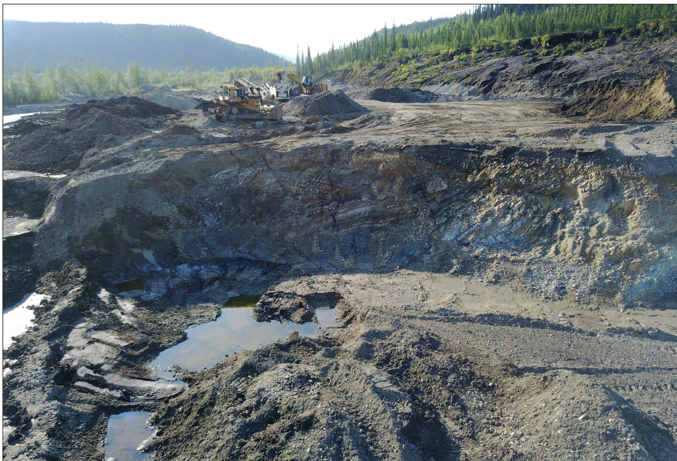
Figure 8. The bedrock exposure on the low-level Hunker Creek bench targeted by Ace Placer Mining Ltd. in 2021.
