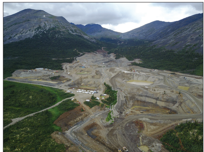
Figure 14. View looking up Granite Creek valley with Dulac Mining's cut in the foreground.
