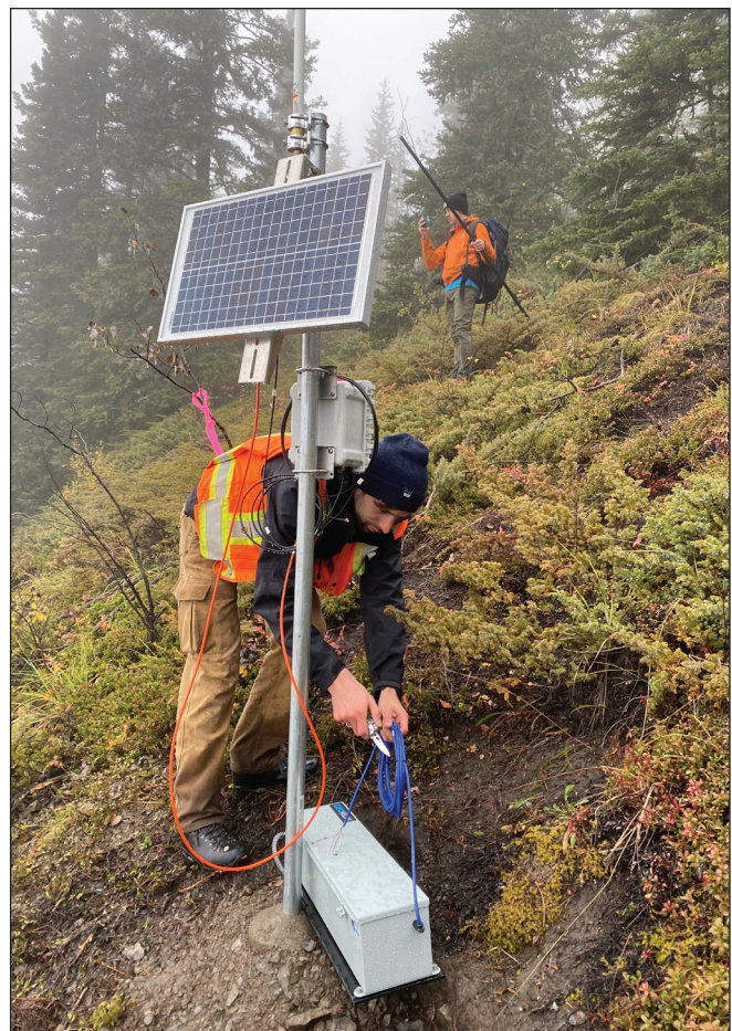
Figure 7. BGC Engineering staff installing an extensometer on the Moosehide Slide in September, 2022.
