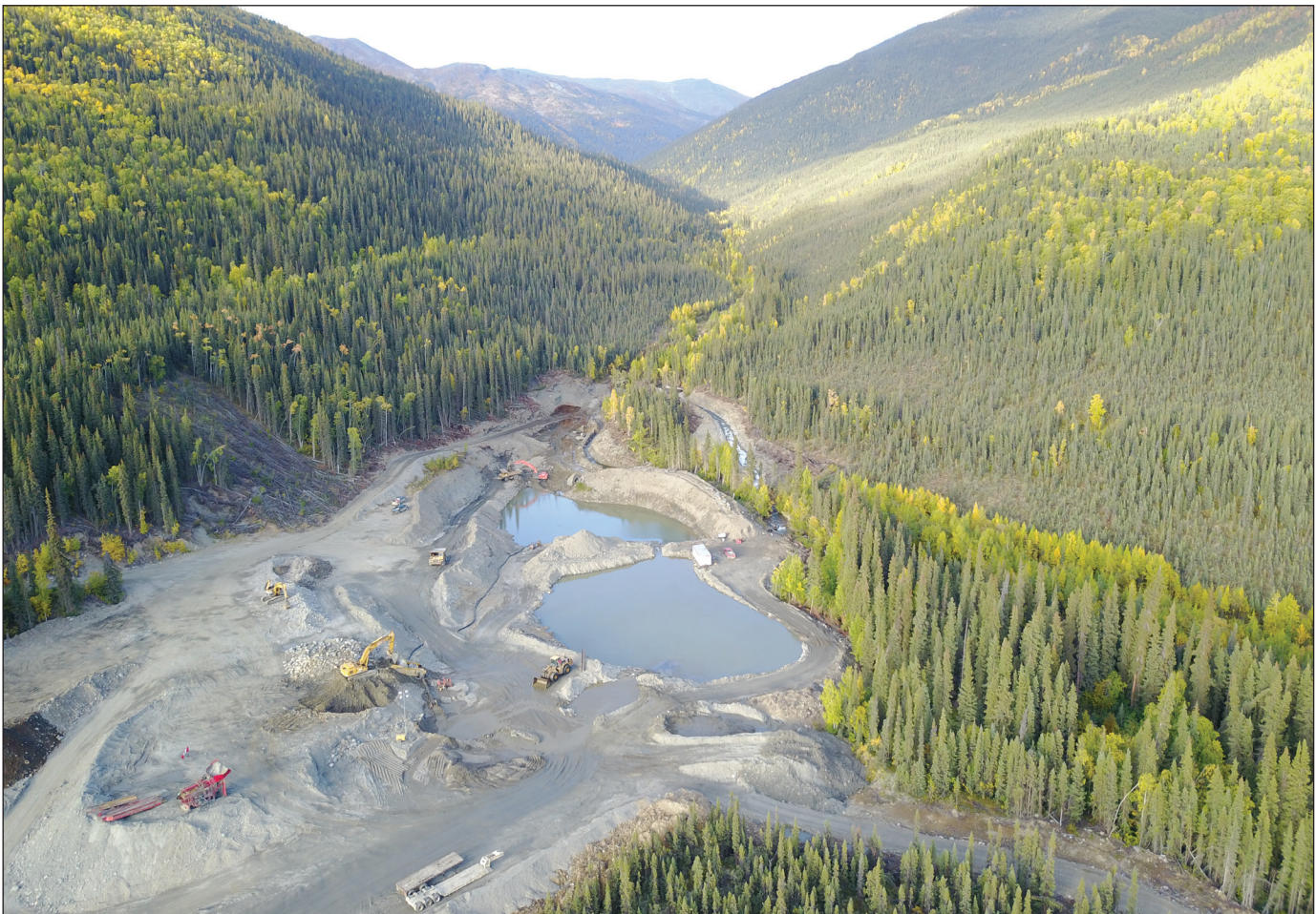
Figure 15. A view looking upstream on Keystone Creek of Dulac Mining's operation.
