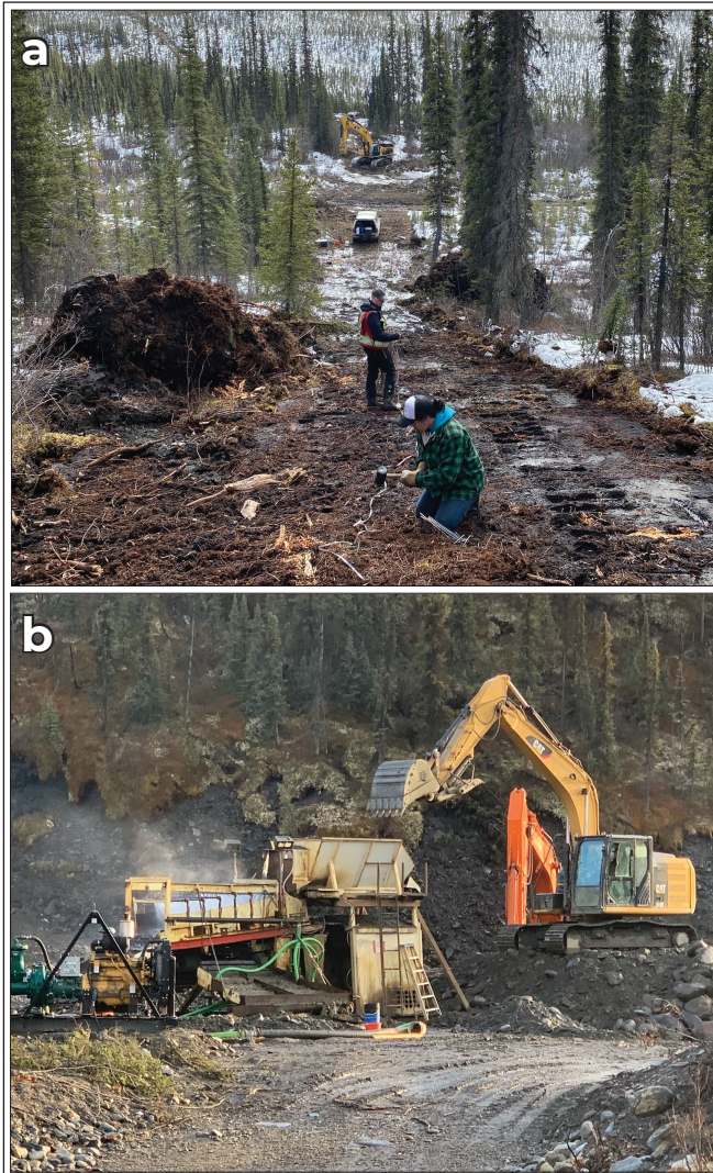
Figure 5. (a) IP survey and (b) bulk sampling on Lightning Creek.
