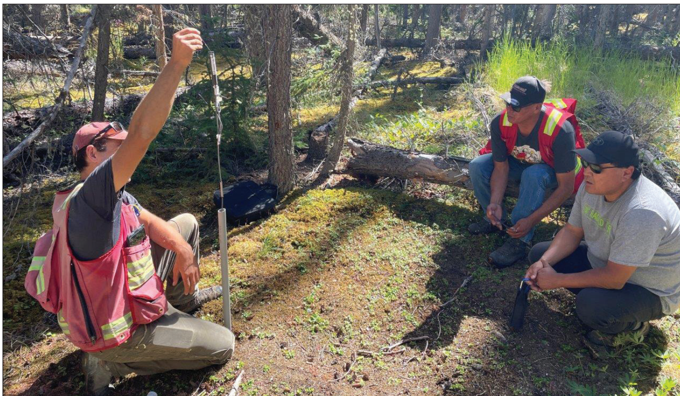
Figure 8. Derek Cronmiller installing a thermistor in a borehole. This one of four instrumented boreholes established in the Haines Junction area to monitor permafrost.
