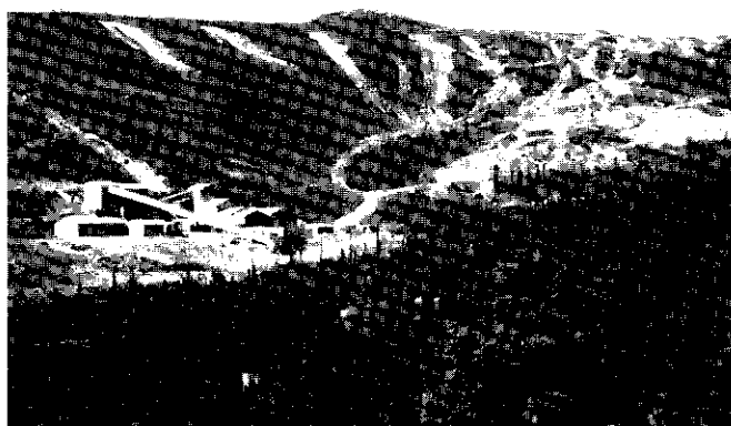
Figure 11: The mill at the Mt. Nansen mine is being upgraded to 700 tonnes per day and a carbon in pulp cyanide circuit added. The Huestis vein that was a focus of exploration in 1995 is located behind the mill.
