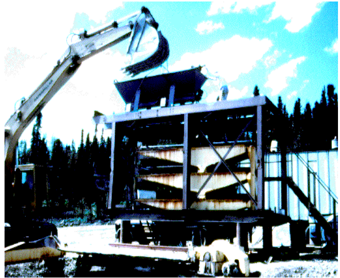
Figure 9: Sikanni Oilfield Construction installed a plant to process high grade gold vein material on its Claymore property in the Moosehorn Range.
