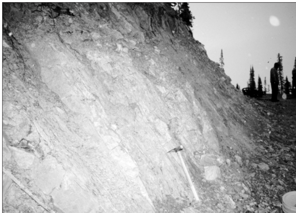
Figure 20. Limonitic-altered quartz sericite schist outcrop on Lake Creek at the Livingstone Creek property northeast of Whitehorse.
