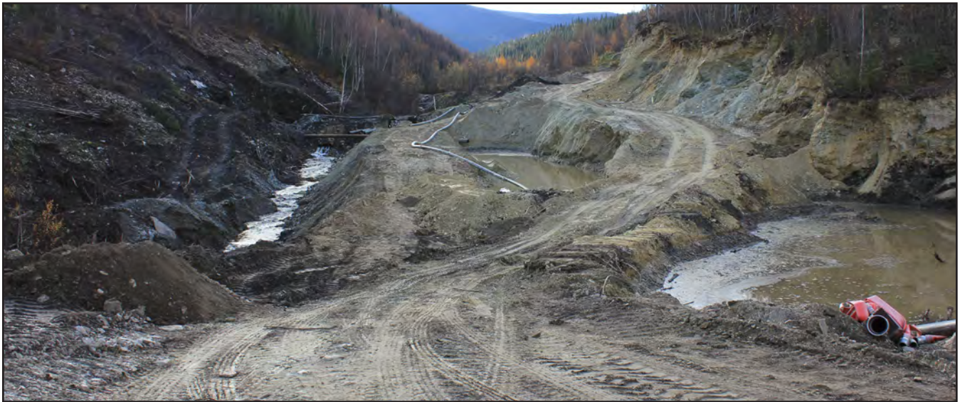
Upstream view in 2014 of the Gardiner's operation on Adams Creek.
