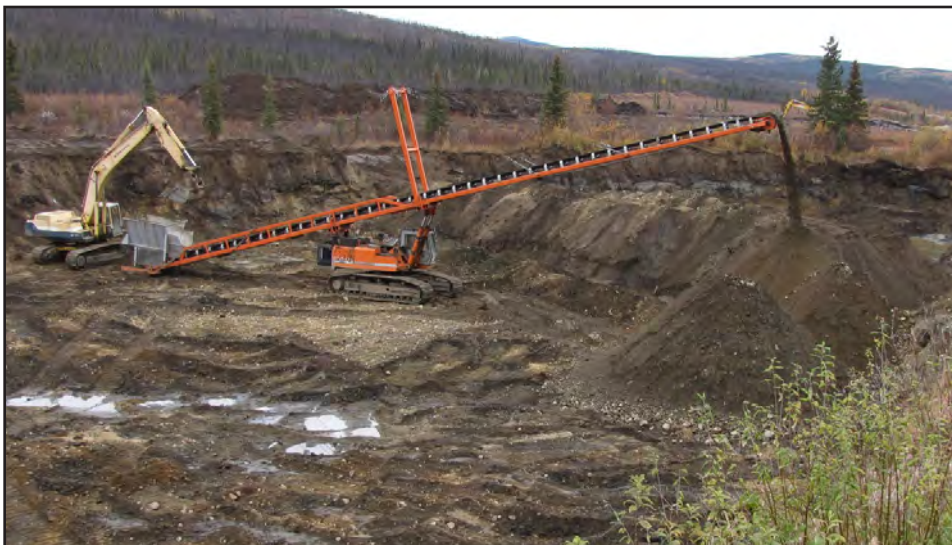
Mr. Hollis' operation on Dominion Creek in 2013, showing his custom-built track mounted conveyor.
