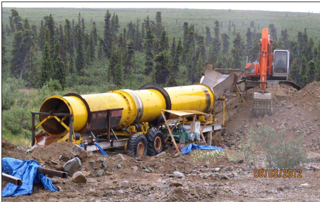
Canaan Gold Resources Inc. wash plant in 2012. (Photo credit: Steve Beaulieu).
