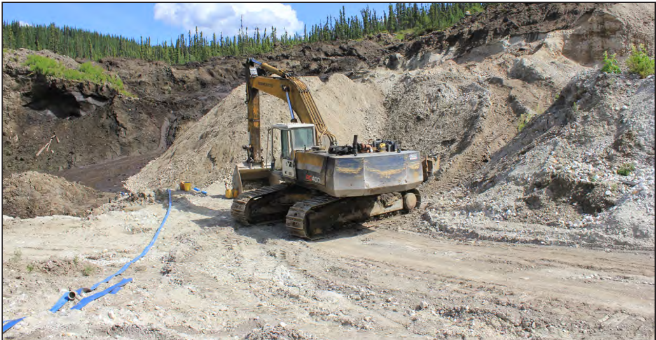
Mr. Brickner's active cut on left limit Lovett Gulch in 2014.
