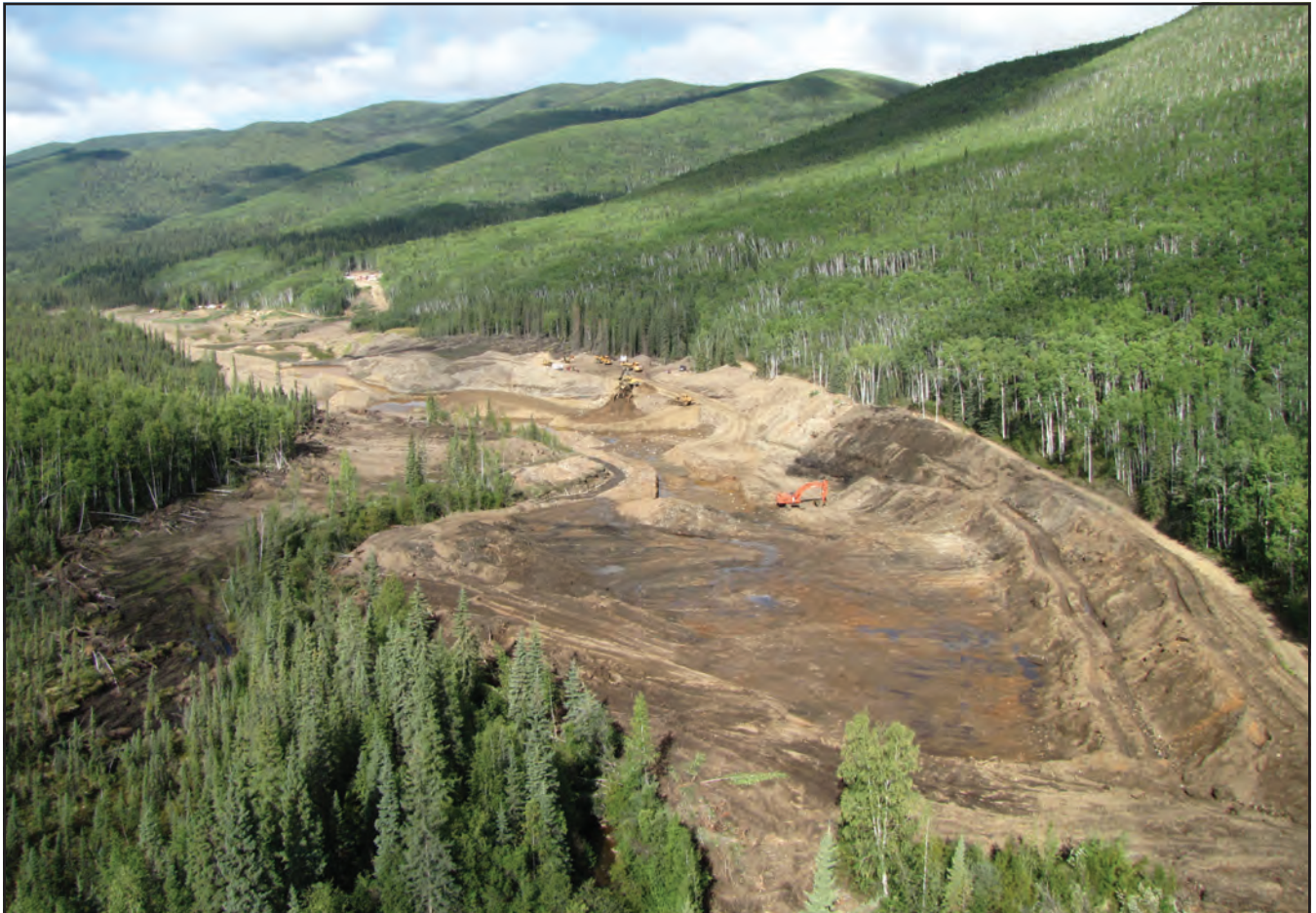
View looking west (downstream) of the Sager operation on Kirkman Creek in 2014.
