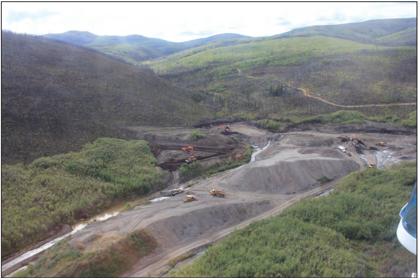
Paydirt Holdings' operation at the forks of Black Hills Creek in 2014.
