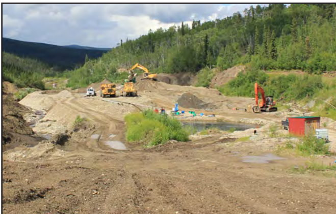
Downstream view in 2014 of the Rodal Placers operation on Eldorado Creek.
