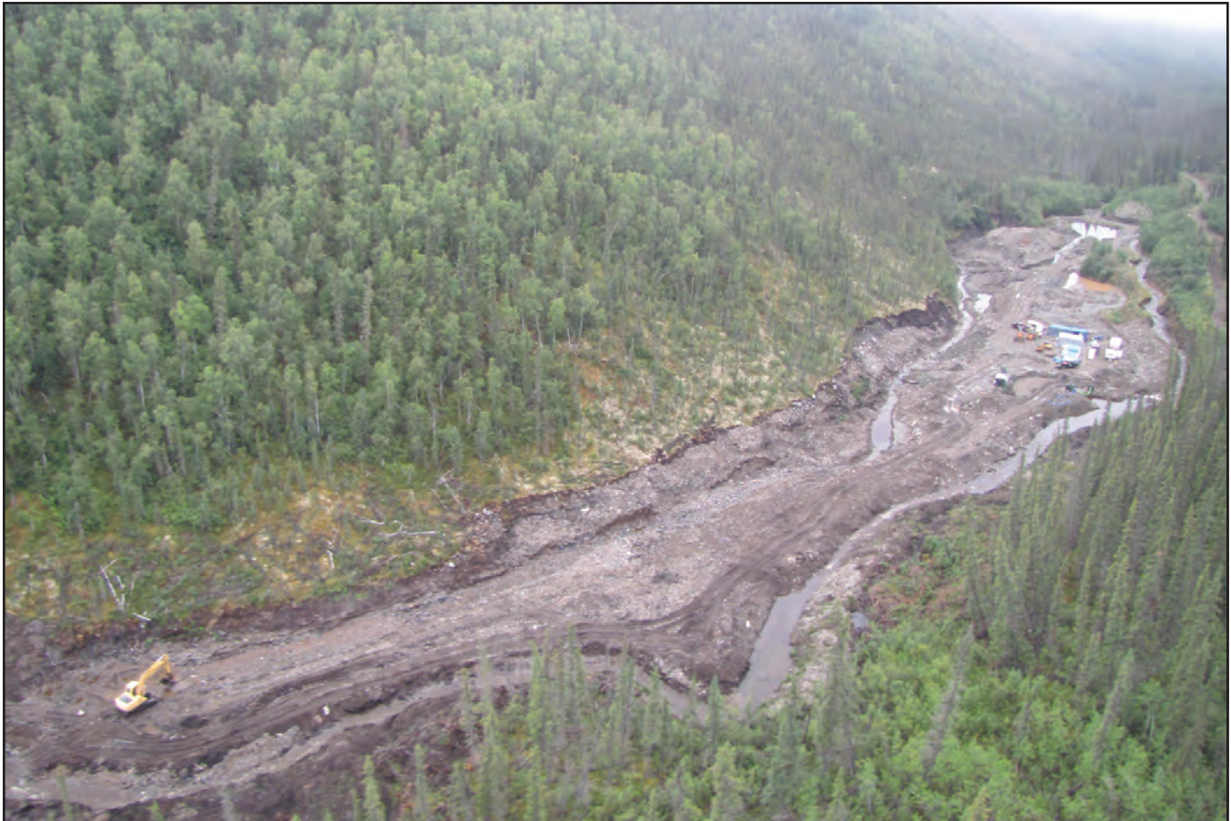
A view down valley of New Age Drilling and Mining's operation on Frisco Creek.
