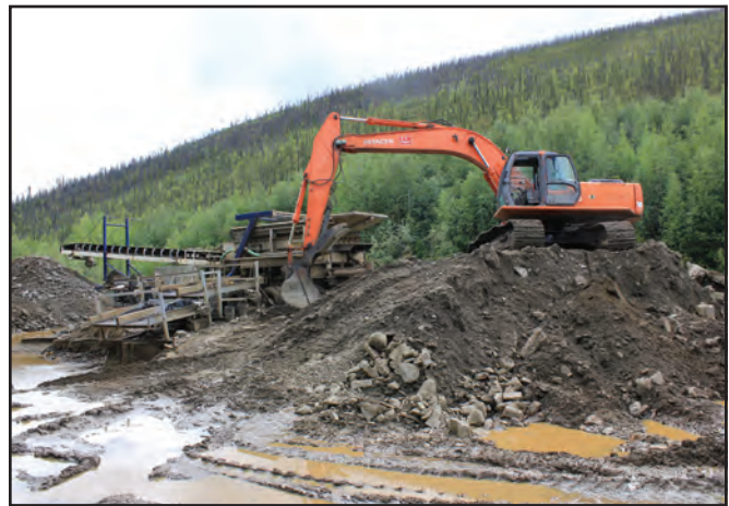
Mr. Neudorf's wash plant in 2014, mining under PM10-071.
