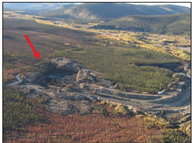
View to the northwest looking over Northern Exposure's left limit cut (see arrow) on Kathleen Creek in 2014. The Indian River is in the background.
