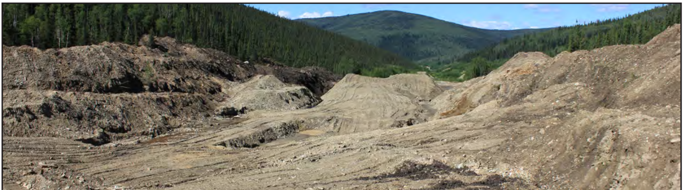
Downstream view of activity from the mouth of Ready Bullion Gulch.
