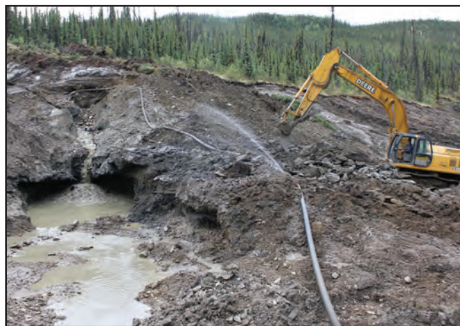
Mr. Minelli stripping and preparing ground in 2014, operating under PM11-052.
