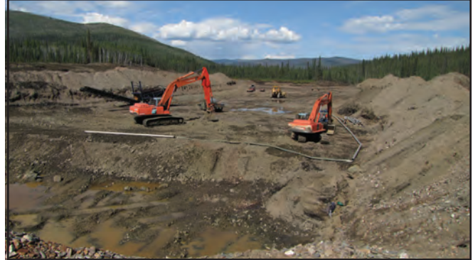
The Hambrook's operation located along Black Hills Creek on 2011, looking upstream.
