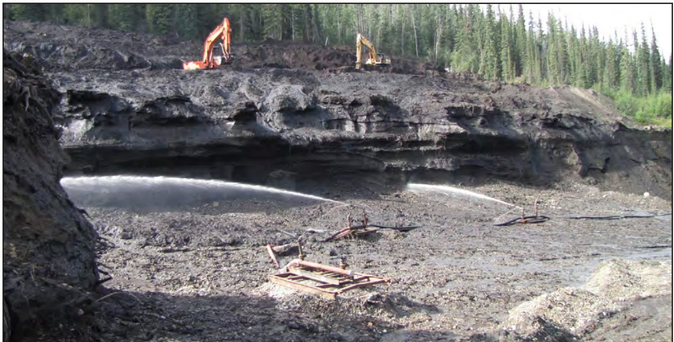
A view of the left limit bank of Independence Creek. The thick muck section was removed using irrigation sprinklers and mechanical excavation.
