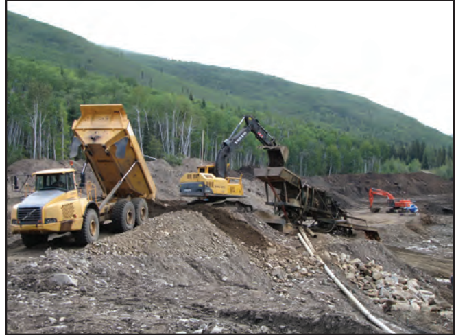
The Sager's mining operation on Kirkman Creek in 2014.
