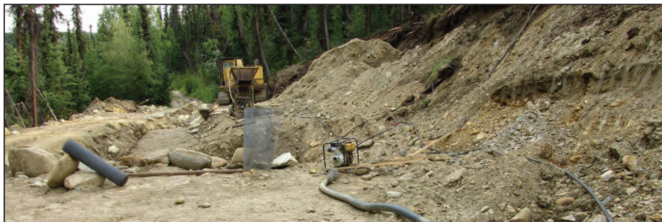
McIntyre Creek cut along the access road in 2013.
