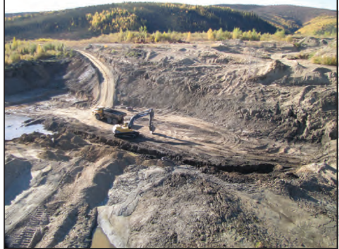
View to the south of Magna North's upstream cut on the right limit of Matson Creek in 2014.
