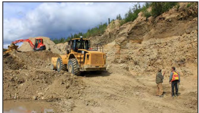
Mr. Nibbecker's bench cut in 2014, on the right limit of Bonanza Creek.
