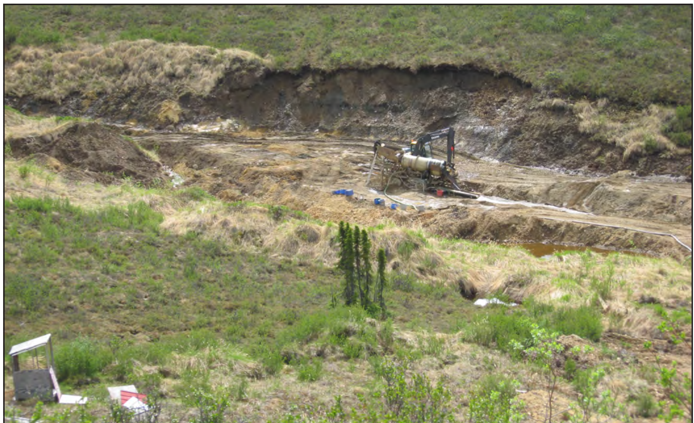
Wash plant on Discovery Creek under PM04-410-2 in 2011 (Photo credit: Steve Beaulieu).
