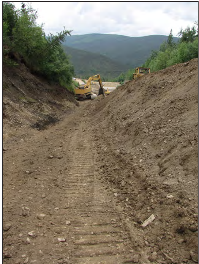
A view looking downstream Oro Grande Gulch towards the active mining area and wash plant.
