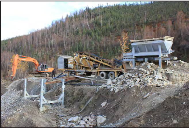
The Gardiner's wash plant in 2014.
