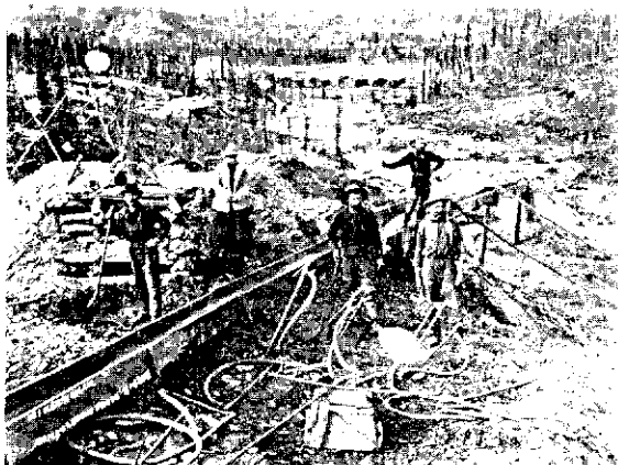
Typical Placer Operation: Happy Gulch-Hunker Creek circa 1903 with shaft and windlass and sluice boxes, thawing equipment in foreground. (Yukon Archives—Adams, Larkin and Cantwell Collection)
