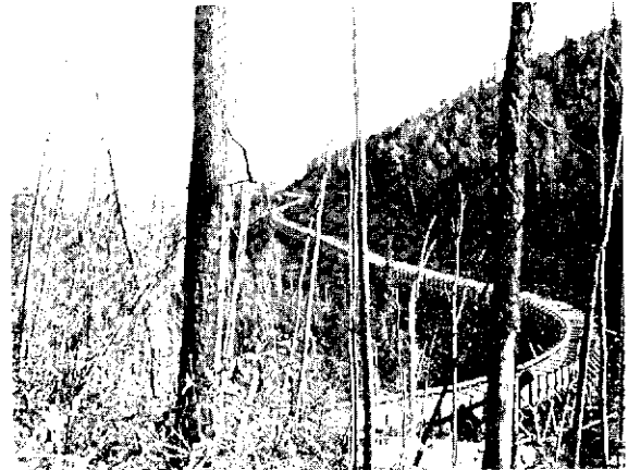
The Yukon or Twelve Mile Ditch: A section of 6 foot by 4 foot flume, part of the 70-mile aqueduct, in 1908. (Yukon Archives—Schellinger collection)
