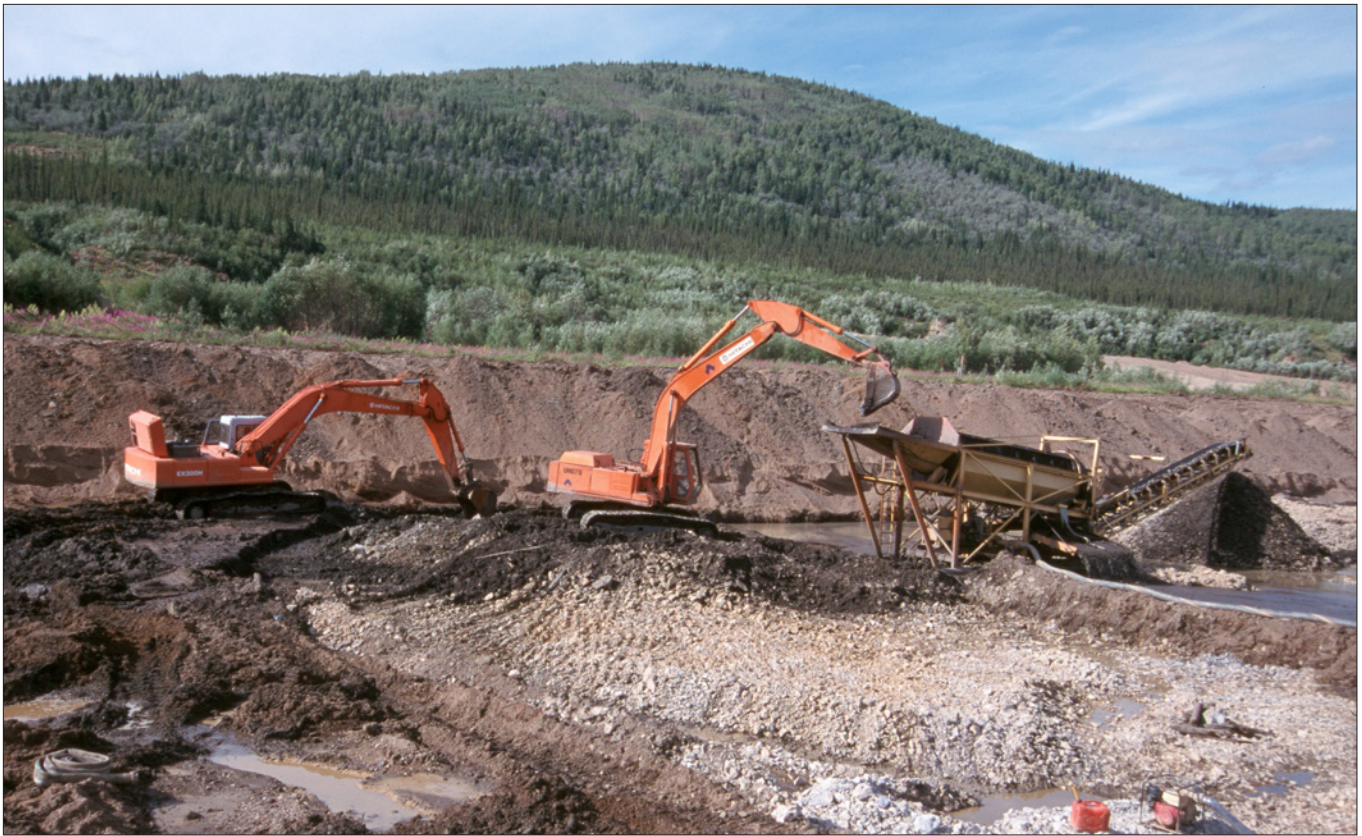
Figure 5. On Sixtymile River, dredges were unable to completely clean the undulating bedrock surface. Pockets of economic virgin gravel were left behind and buried under dredge tailings, waiting to be re-exposed by today's placer miners.
