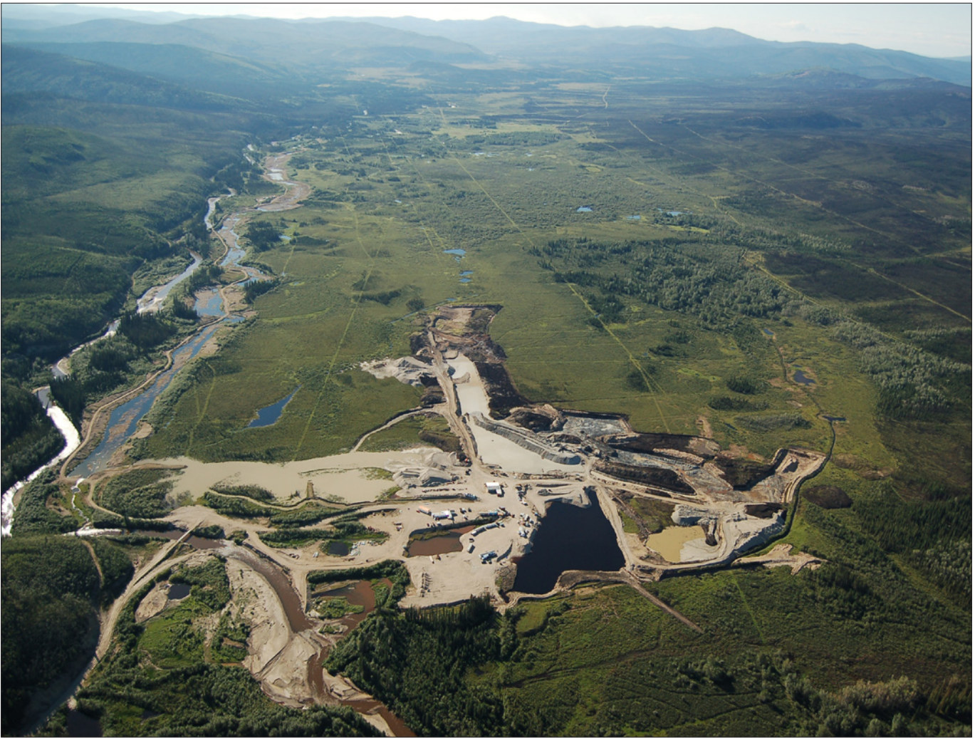
Gimlex Enterprises Ltd.'s mining operation on Indian River in 2006; view to the east.
