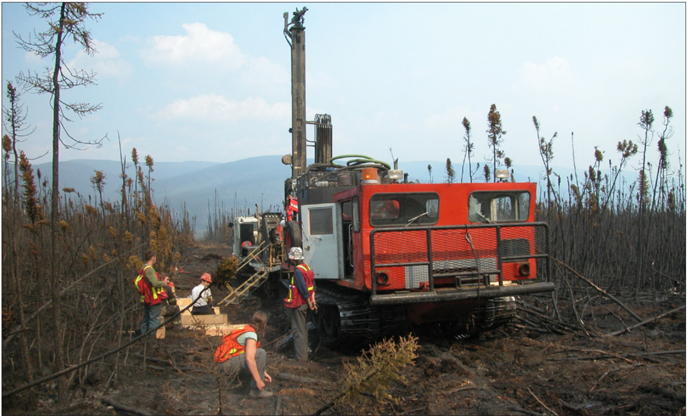
Boulder Mining's rotosonic drill on Indian River, 2004.
