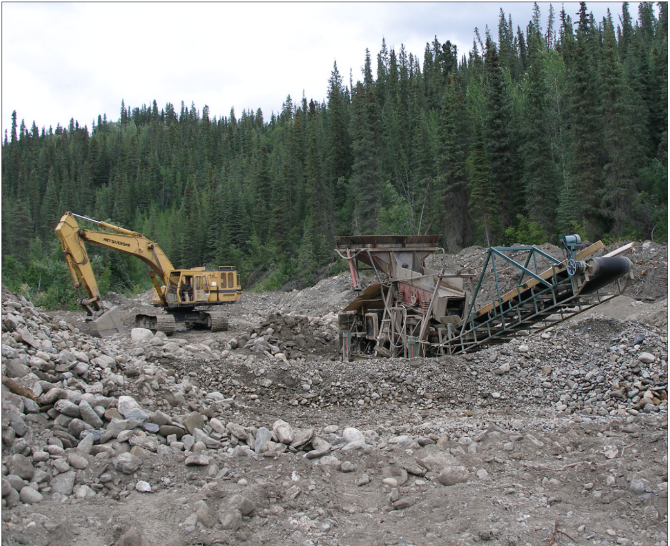
Gateway Explorations' wash plant above the falls on Iron Creek, 2006.
