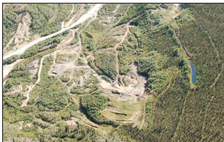
Aerial view of Ralph Troberg's operation on the left limit of Bonanza near Boulder Creek, 2008.
