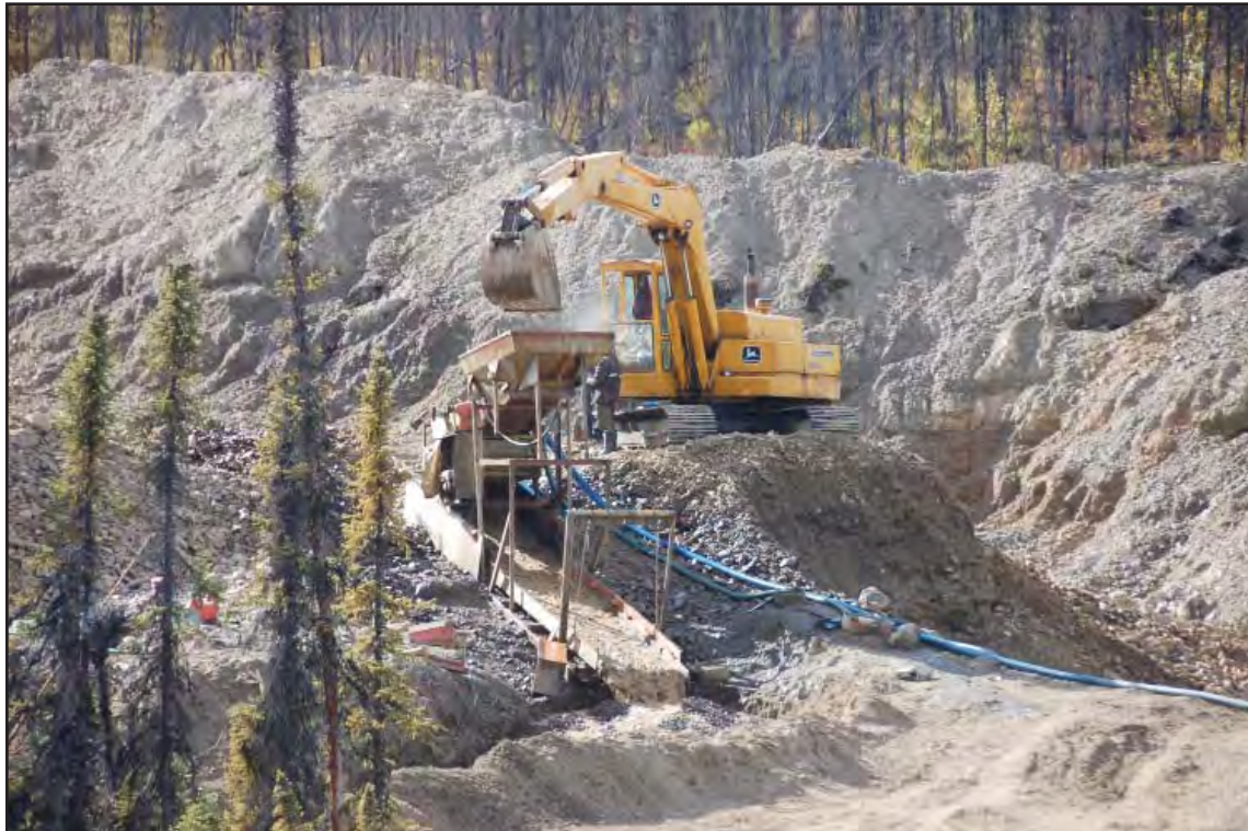
Ripper Mining on upper Eureka Creek in 2008.
