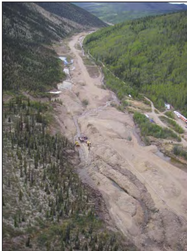
Blackstone Placer's mining operation on the Left Fork of Clear Creek in 2008.
