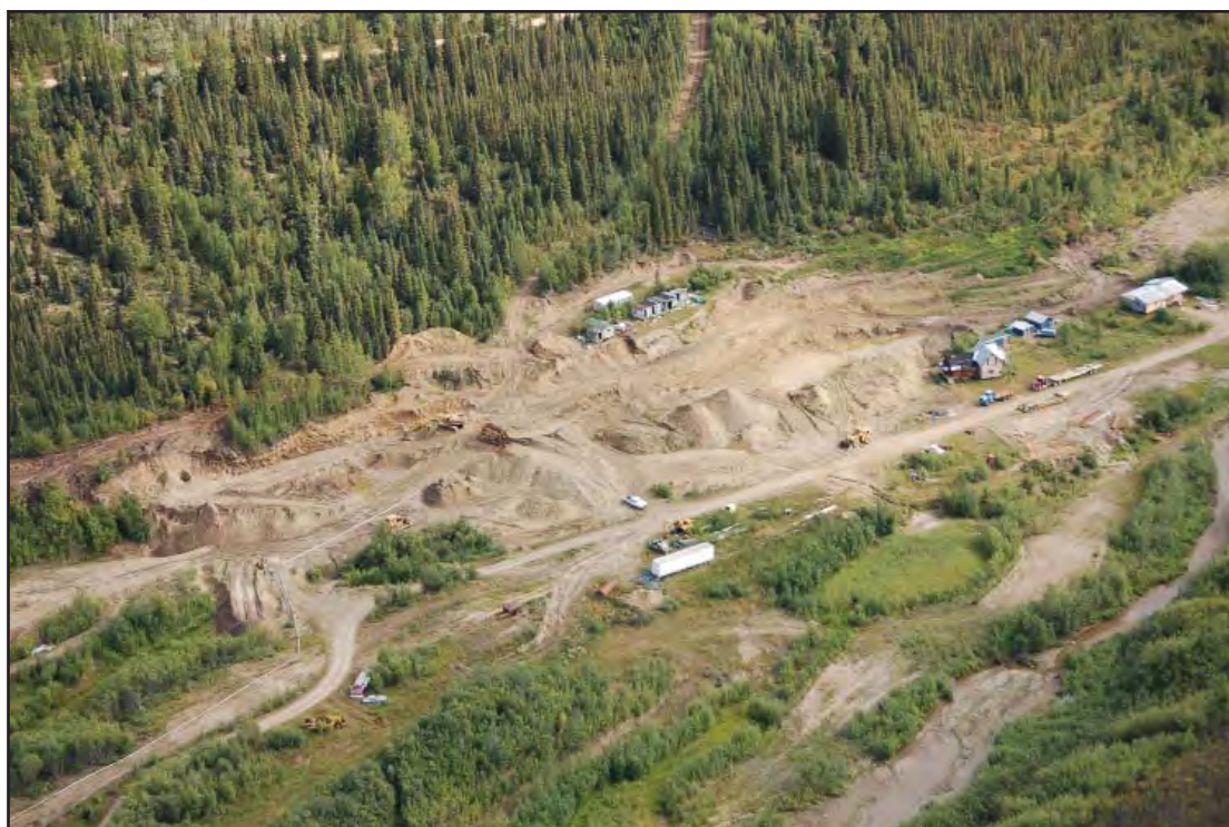
Aerial view of Dan Klippert's downstream mining cut on Sulphur Creek in 2008.
