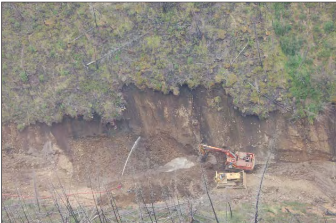
Hydraulic monitoring at Mike Ward's mining operation on Boliden Creek in 2007.
