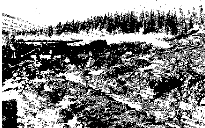
Hydraulicking to remove black muck from the D. Gritzka property along Sulphur Creek during 1982. A bulldozer was also used for stripping.
