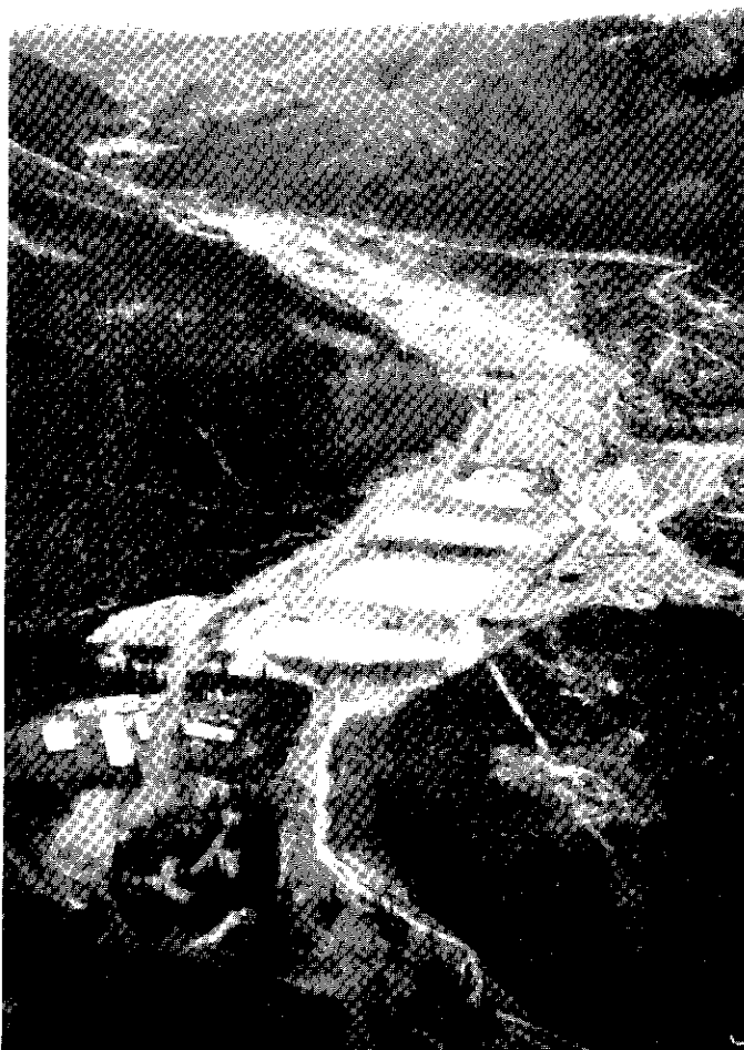
View upstream along Dublin Gulch at the Canada Tungsten Mining Corp. Ltd. property. Four settling ponds and the camp are in the foreground. The mining area and processing plant are in the centre of the photograph. Potato Hills are visible in the background. The Dublin Gulch lode gold occurrence lies in the centre distance of this scene. The Ray Gulch tungsten deposits lies to the right (south) of the photograph.
