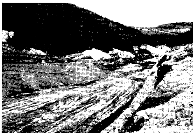
Mining at Arctic Rim Operators property along Bear Creek. Scraper-loaders were used to work in the long, narrow cuts at this site.
