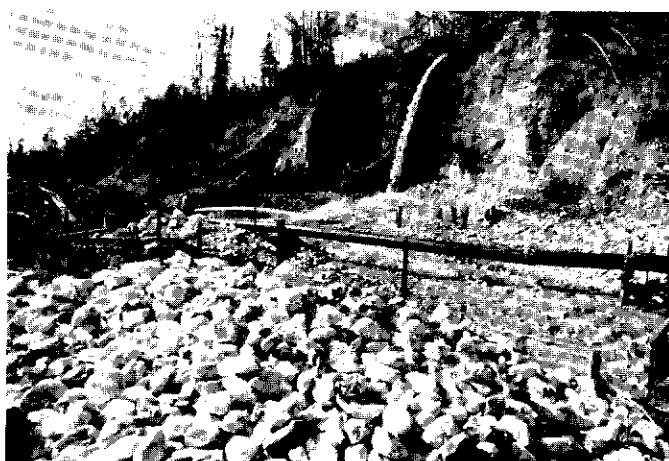
Hydraulic mining at the I. Bremner property on Bryan Bench of Last Chance Creek. Large boulders in the foreground were picked from the gravel and stacked by hand. The head of the sluice box set in the floor of the cut is visible at lower right.
