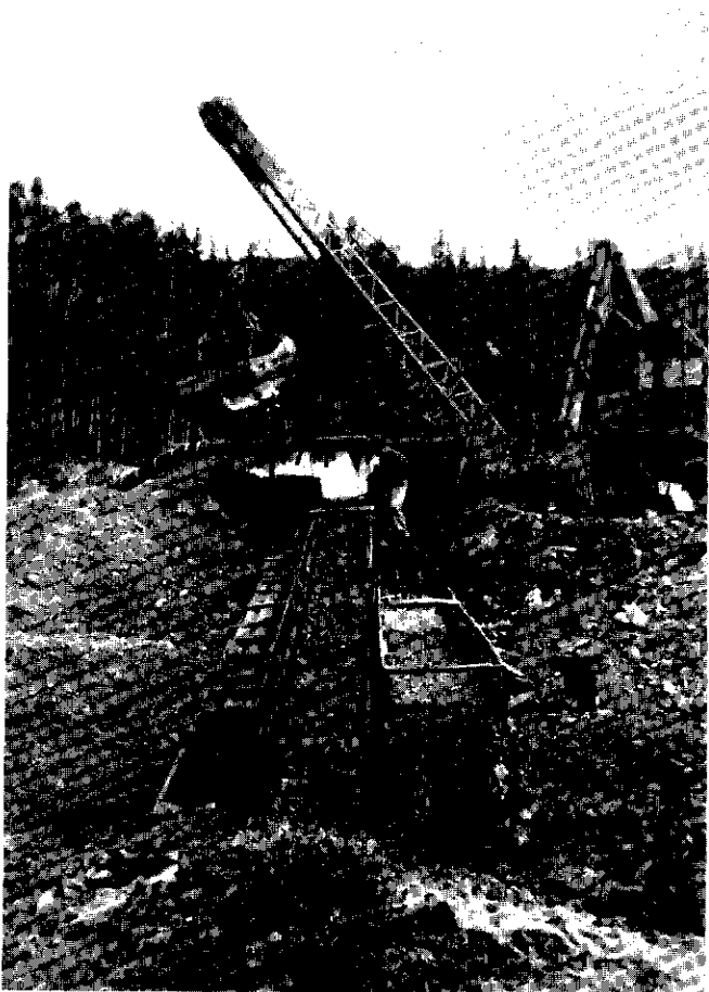
Figure 19: Dragline feeding sluicing plant at W. Hinnek mining operation on Bonanza Creek. (R.W. '84)
