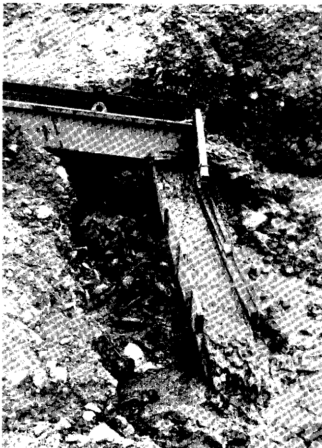
Figure 5: Small side run at the end of the main sluice run set up by Dublin Gulch Mining to recover fine grained gold at the Chumar Placers property on Miller Creek. (R.W. '84)
