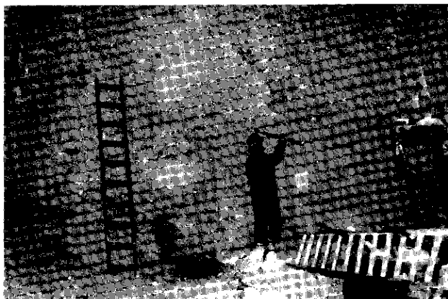
Figure 2: Loading rounds for blasting at Jackson Hill mine of White Channel Underground Mining Ltd. (C.M. '84)
