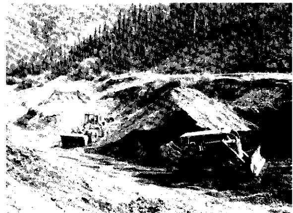
Looking downstream on French Gulch at a Caterpillar D8K bulldozer and 980 front end loader belonging to Jim Archibald.
